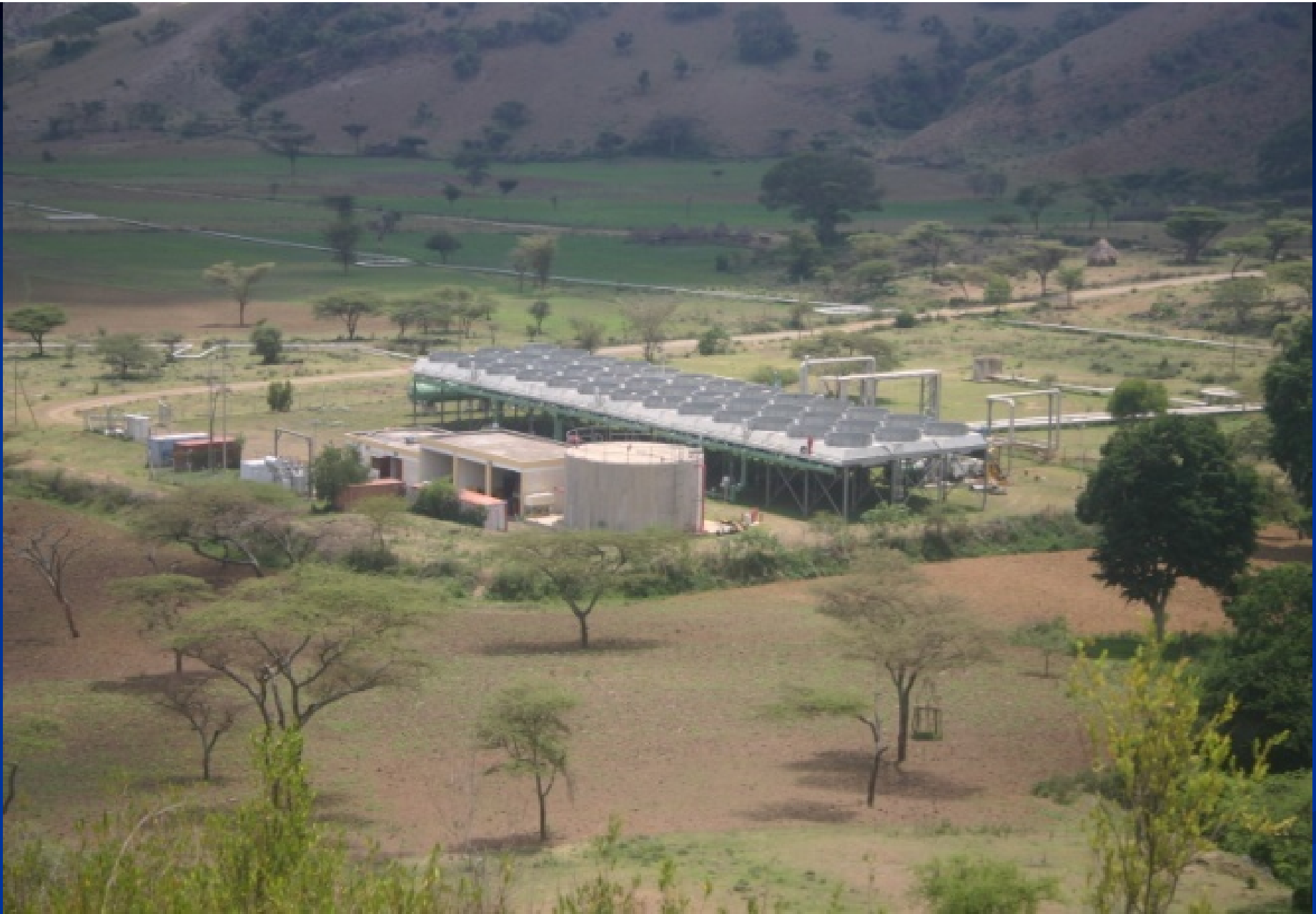
The Aluto Geothermal Pilot Power Plant
